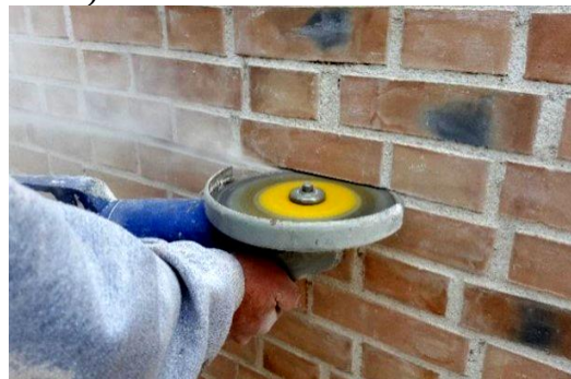
2-rasm. Bog'lanmagan choklarni parmalash orqali ochish
