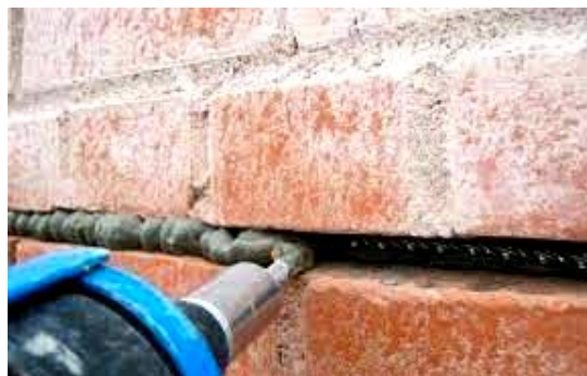
4-rasm. Po'lat simni yelimlash jarayoni
