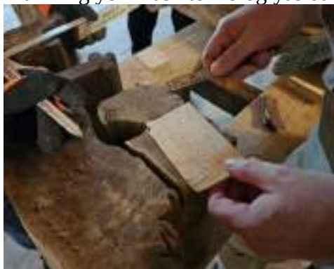
1-rasm. Xivadagi "Juma Machit" yodgorligining yog'och ustunlarini yelimlash jarayonlari
