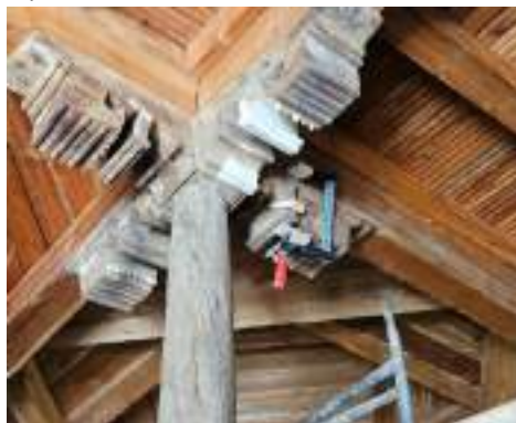
1-rasm. Xivadagi "Juma Machit" yodgorligining yog'och ustunlarini yelimlash jarayonlari
